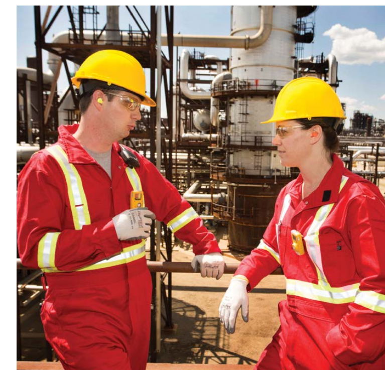
Workers climb stairs within the Quest unit at the Scotford Upgrader, near Fort Saskatchewan (northeast of Edmonton), AB in June 2015.
